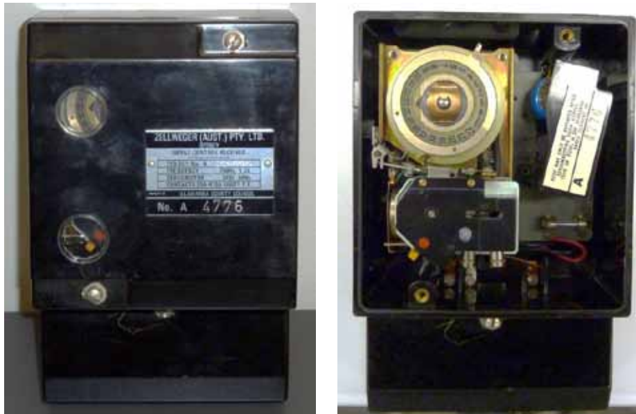
Figure 3.5: Photograph of K22 Receiving Relay with and without Cover
